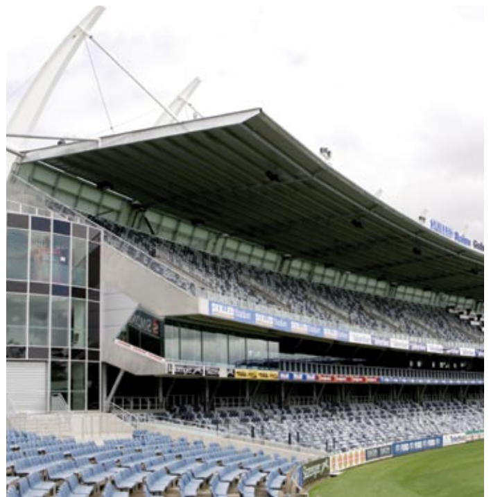
All-weather install at Skilled Stadium, Geelong, Victoria, Australia
